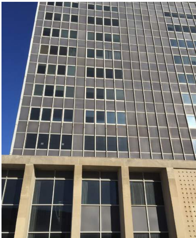
EXISTING BASE AND CURTAIN WALL
